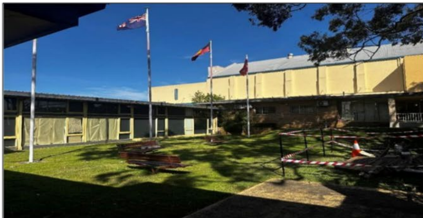
Photograph 2: SSROC Building, as viewed from within the site
