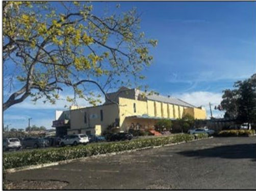
Photograph 7: The rear of Former Orion Theatre, as viewed from within the subject site
