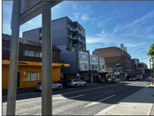
Photograph 8: Shop-top housing developments at Nos. 108-118 Beamish Street, as viewed from Beamish Street
