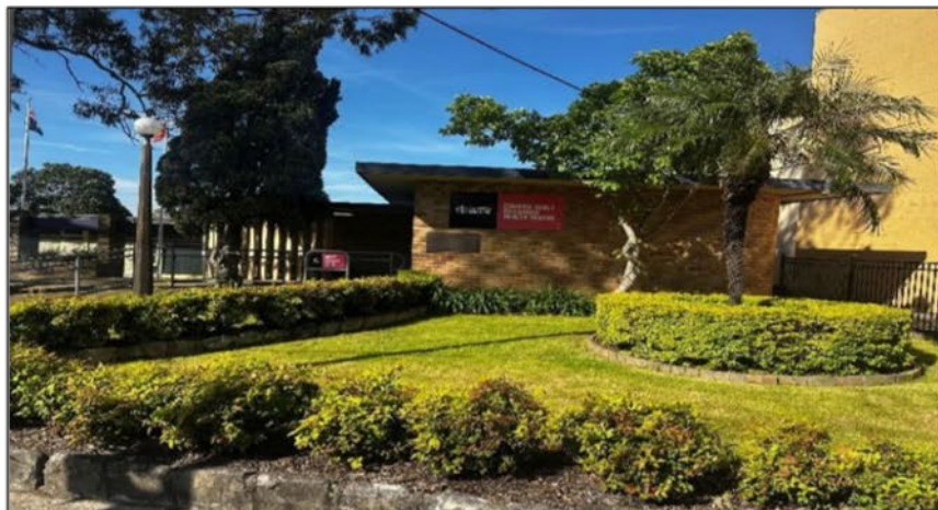
Photograph 3: CECHC Building, as viewed from Beamish Street
